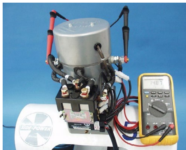
Checking voltage at thruster
